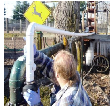
Replacement of an ascending water pipe (green) to a decending water pipe (white) after it was determinend that years of sludge build up supported negative associated organisms in the water.
