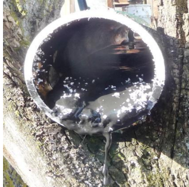
Replacement of an ascending water pipe (green) to a decending water pipe (white) after it was determinend that years of sludge build up supported negative associated organisms in the water.
